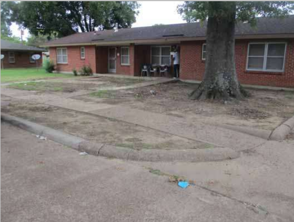
Compliant Accessible Route to Typical Handicapped Dwelling Unit Entry Door, Site 28-1
