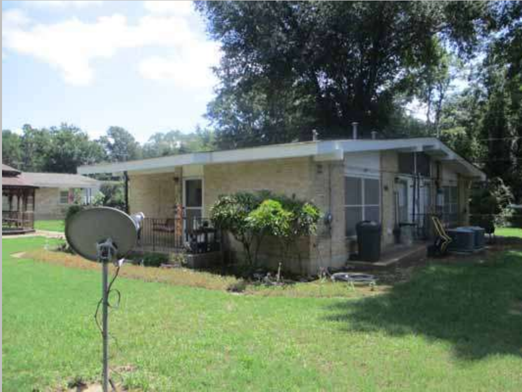
Apartment Building Rear/Side Elevation, Site 28-2
