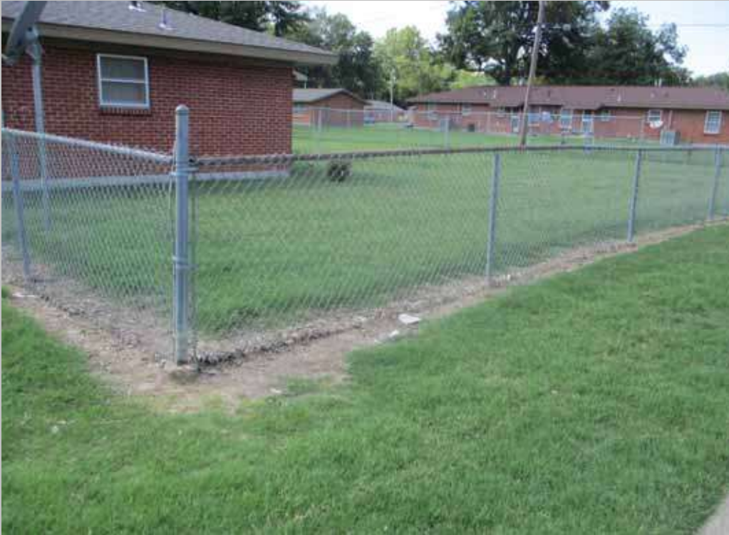
Chain Link Fencing, Site 28-1
