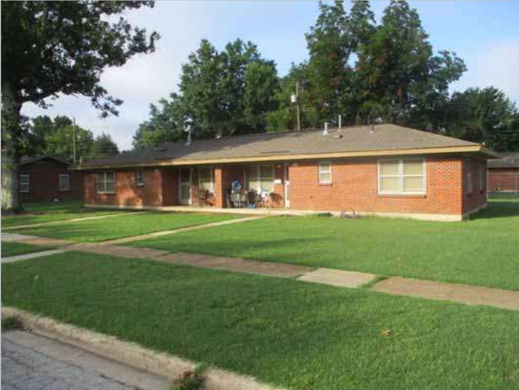
Apartment Building Front Elevation, Site 28-1
