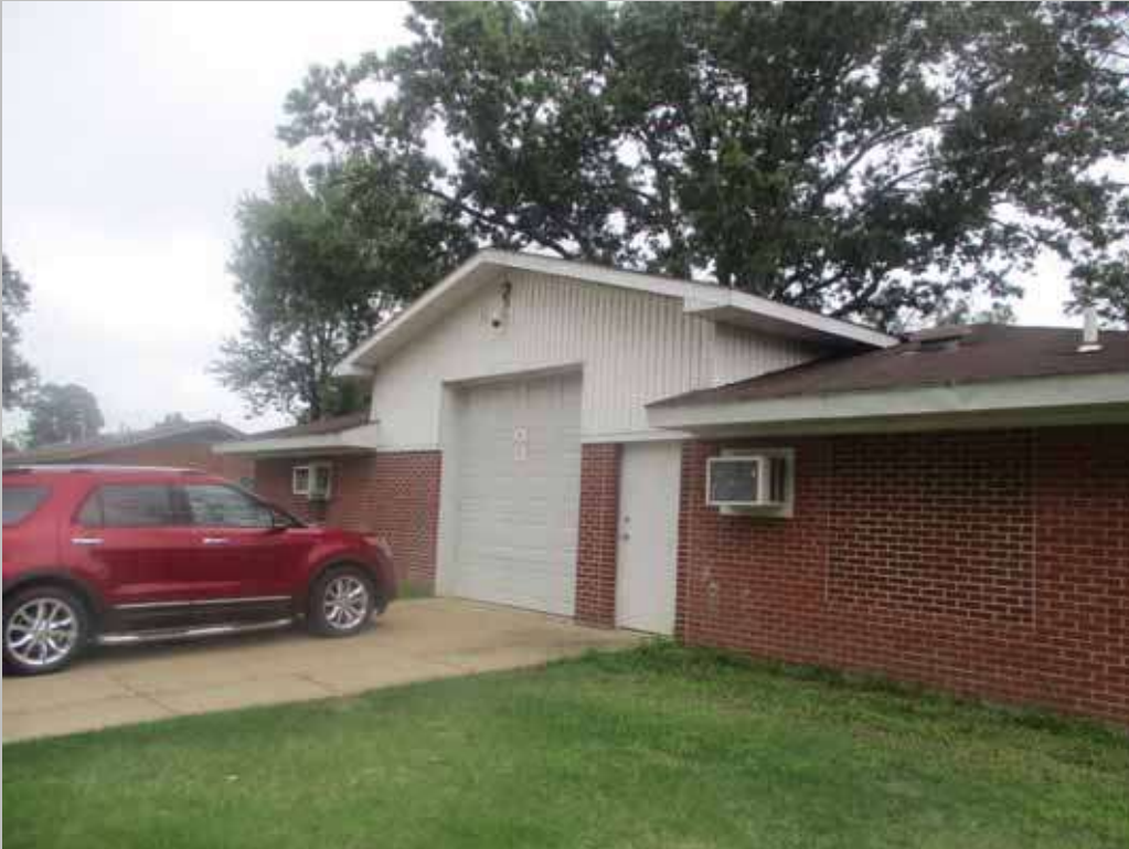
Maintenance Building Front Elevation, Site 28-1
