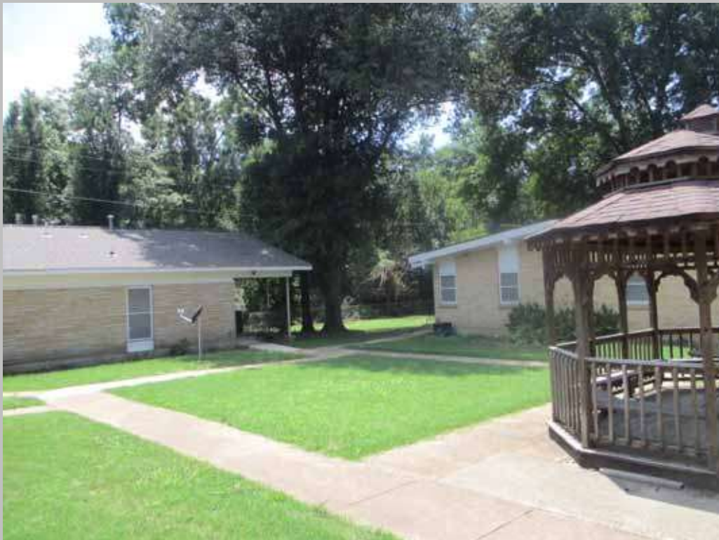
Compliant Accessible Route to Gazebo, Site 28-2
