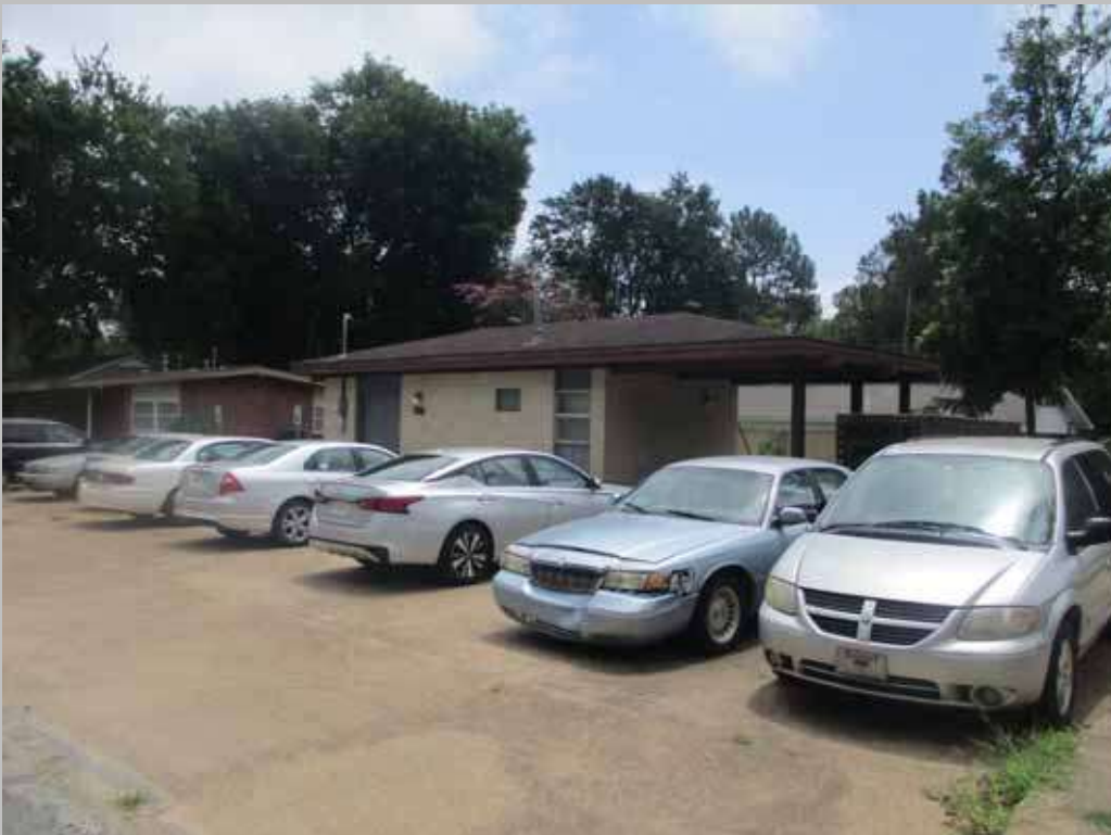
Maintenance Building Front Elevation, Site 28-2
