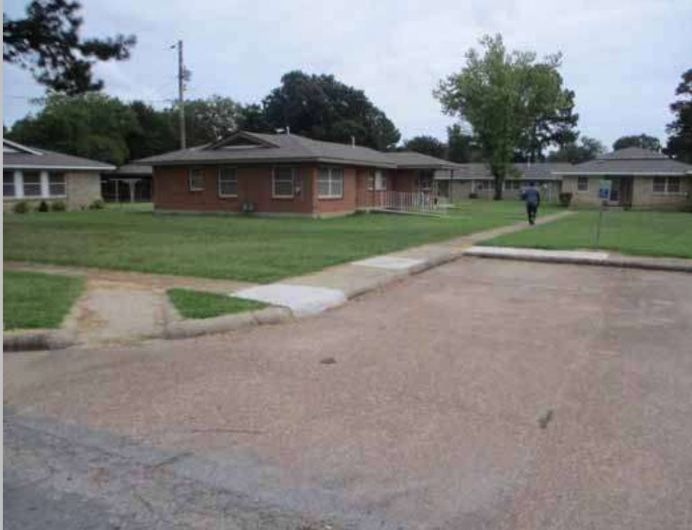
Compliant Handicapped Designated Parking Width, Curb Ramp and Vertical Signage, Site 28-3
