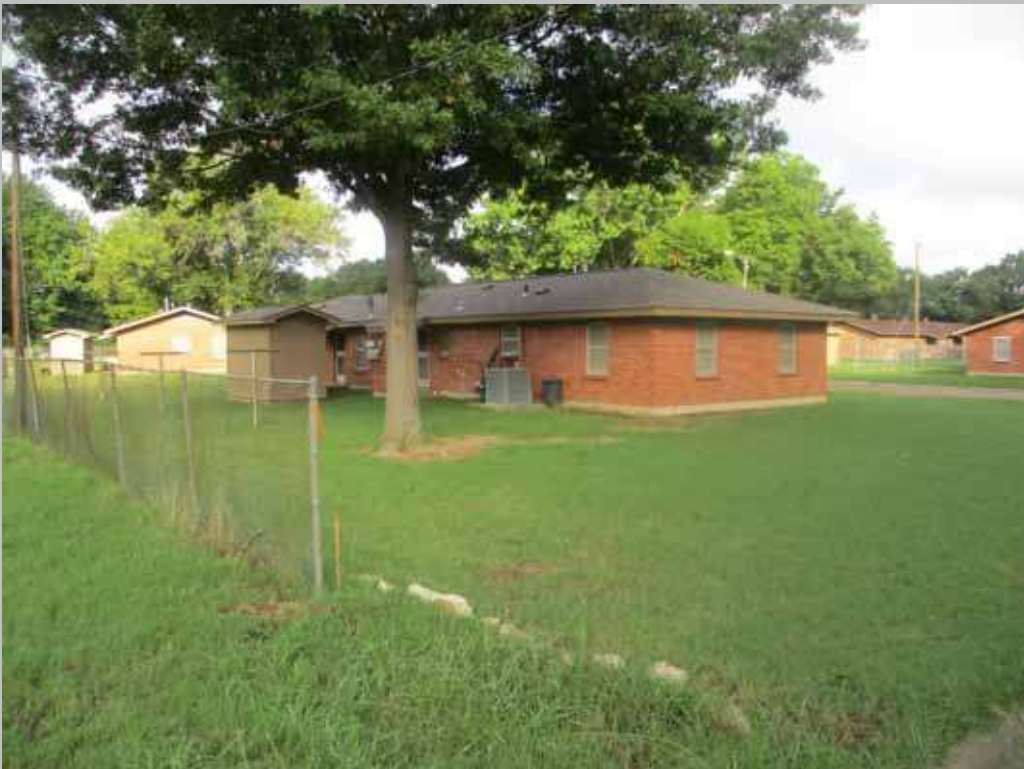
Apartment Building Rear/Side Elevation, Site 28-1
