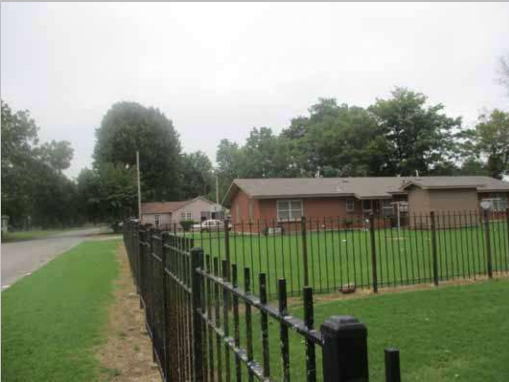
Wrought Iron Fencing, Site 28-1
