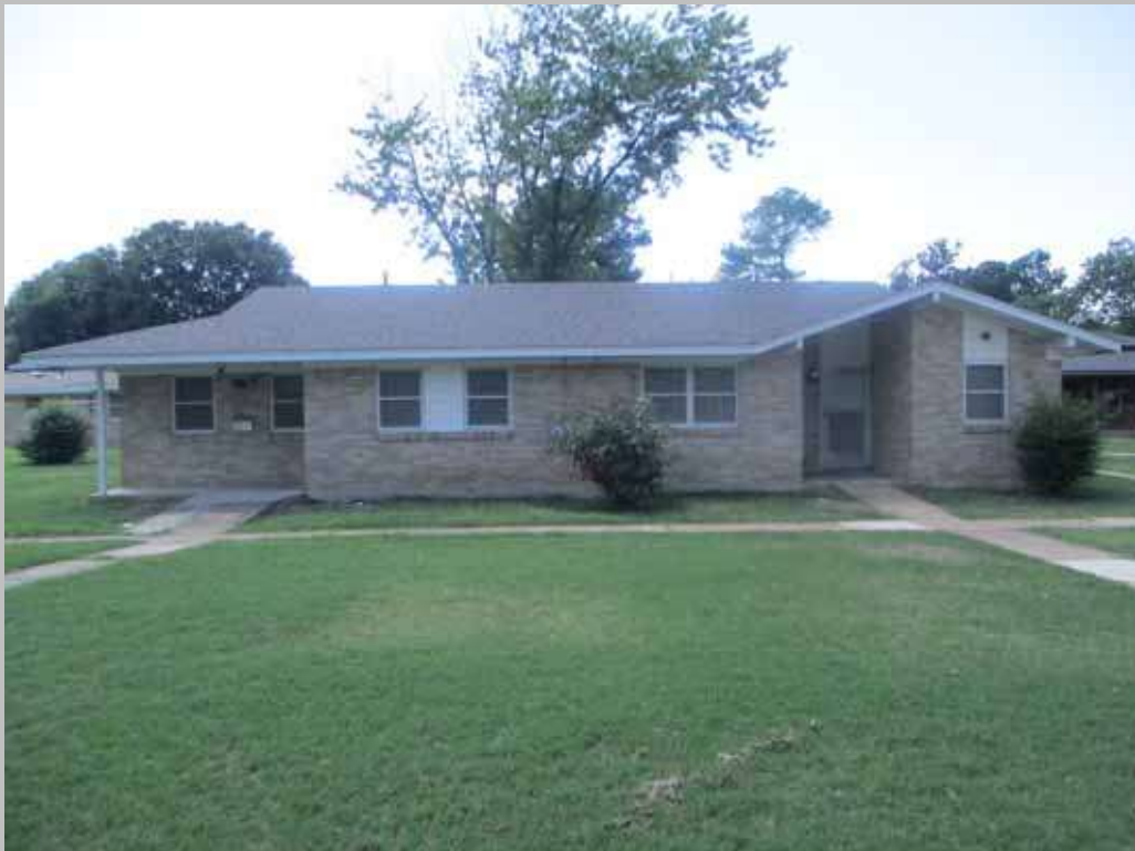
Apartment Building Front Elevation, Site 28-3
