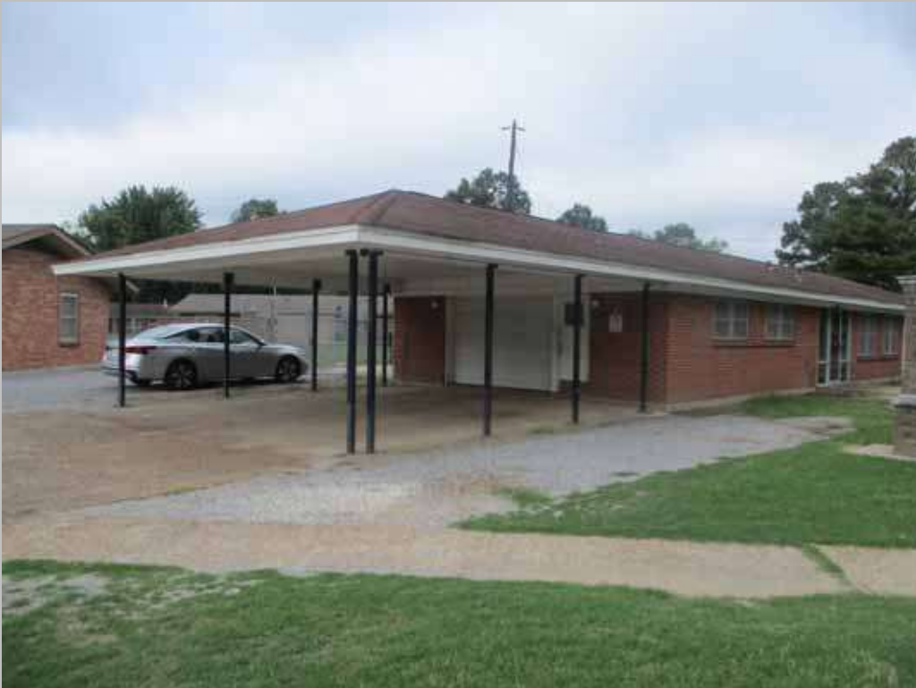
Maintenance Building Front, Side Elevation, Site 28-1
