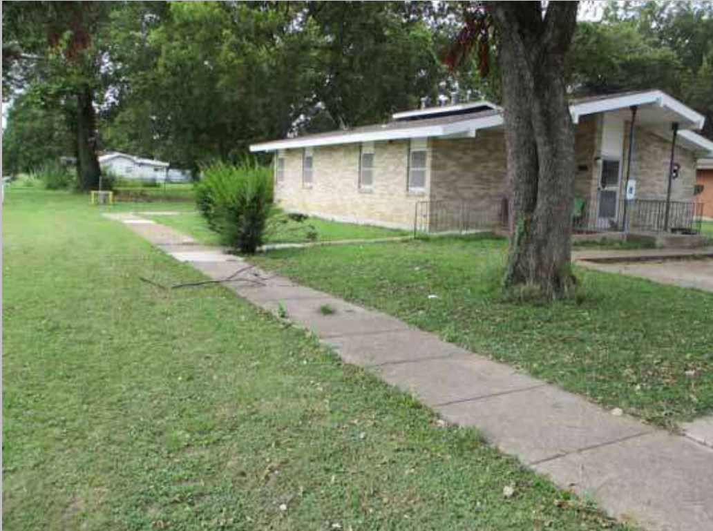
Compliant Accessible Route to Typical Handicapped Dwelling Unit Entry Door, Site 28-2
