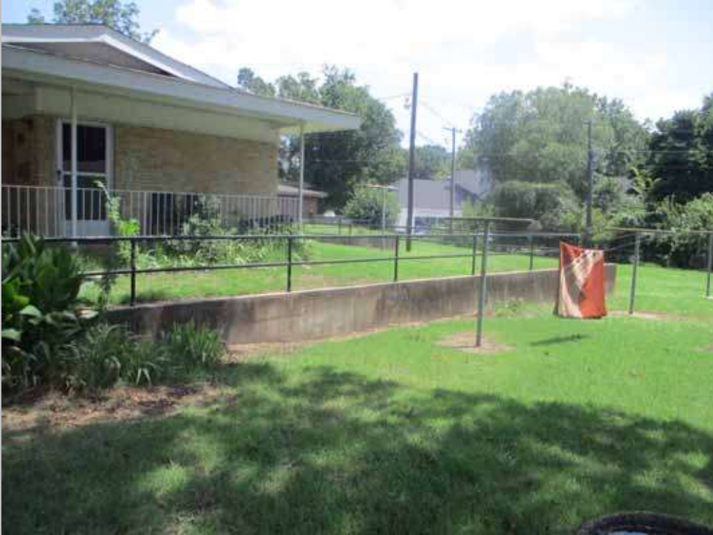
Concrete Retaining Wall, Site 28-2
