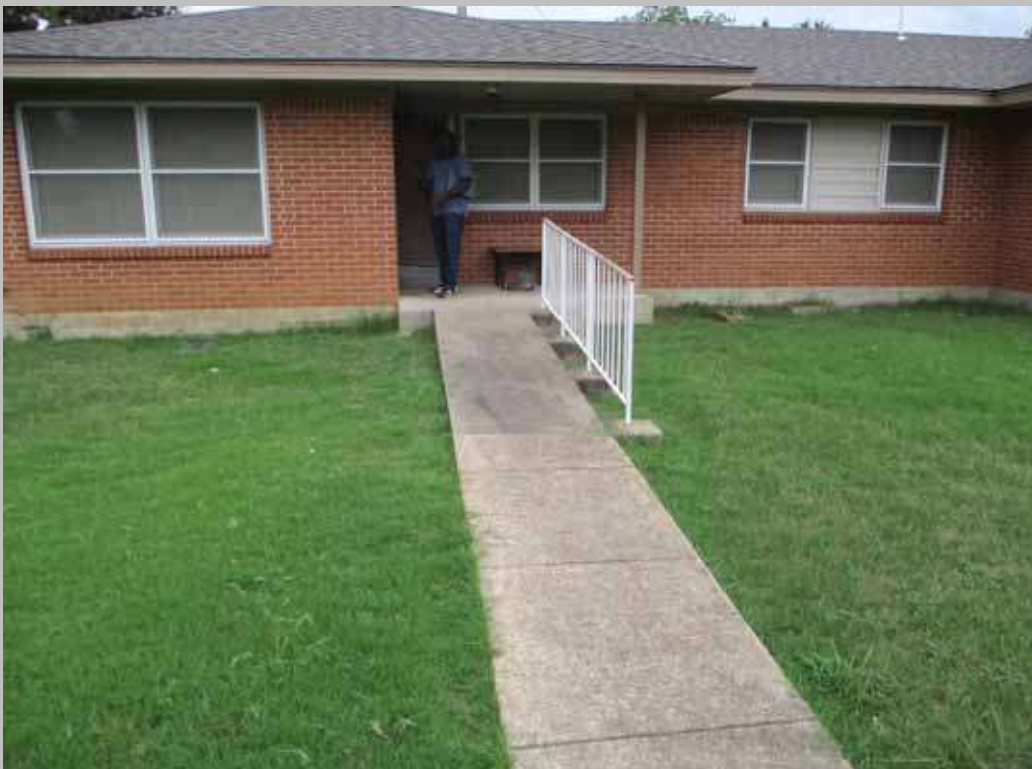
Compliant Accessible Route to Typical Handicapped Dwelling Unit Entry Door, Site 28-3
